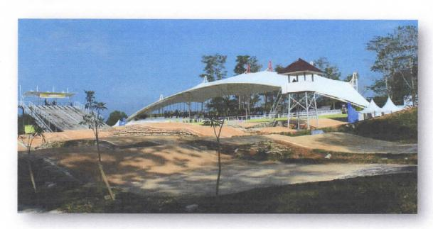
Length of the Track : 345 Meter Height of starting Hill 6,5 meter, there are 3 berms & 2 big jumps.
